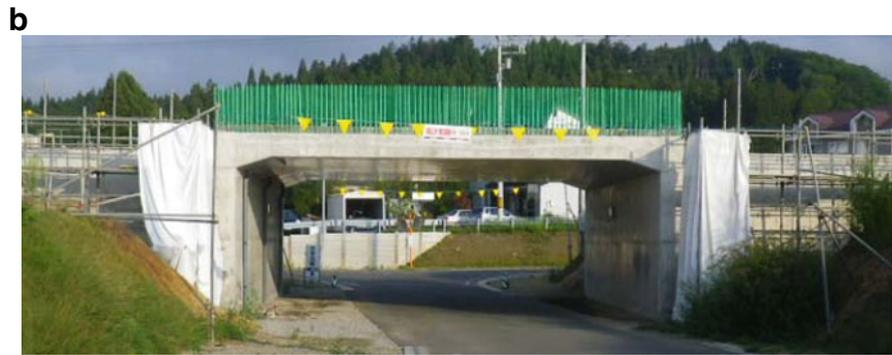
**Fig. 23** GRS integral bridge at Kikonai, Hokkaido Shinkansen (at site I in Fig. 3b)
