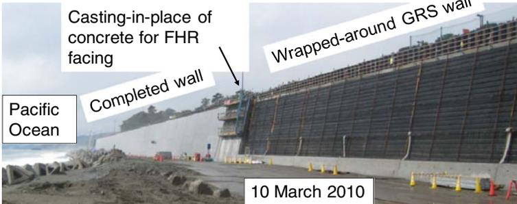
**Fig. 27** **a** Collapse of a masonry RW for the approach fill of a bridge by scouring of the supporting ground, followed by erosion of the backfill by flood, July 2011, and **b–d** restoration to a GRS RW with FHR facing, Iiyama Line, JR East [38]
