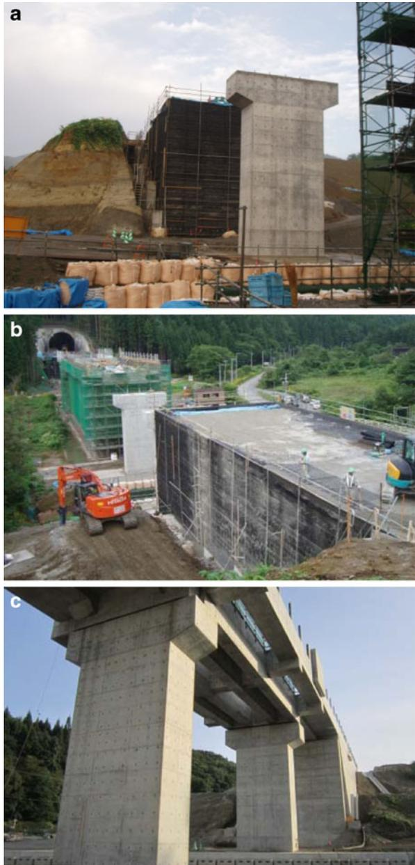
a GRS box culvert in the completed form is different from a GRS integral bridge only in that this has the bottom RC slab. Therefore, the contact pressure at the bottom face of the bottom RC slab of a GRS box culvert is much lower than the one at the facing bottom of a GRS integral bridge. In addition, the bottom RC slab functions as a strut for the facings. Therefore, the stability of a GRS box culvert is higher than a GRS integral bridge under
