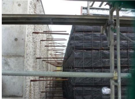
**Fig. 24** GRS box culvert for Hokkaido Shinkansen: **a** general structure; the numbers denote the construction sequence (site B2 in Fig. 3b); and **b** a space between the RC box structure and the approach block before step (3) (site B1 in Fig. 3b) [15, 16]
