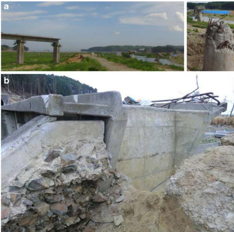
Fig. 34 **a** Tsuyano-kawa Bridge, JR East Kesen-numa Line, that lost multiple simple-supported girders by tsunami forces and **b** a view of the back of the right bank abutment of Yonedagawa Bridge, Noda, Iwate Prefecture, North-Rias Line, Sanriku Railway [44]
